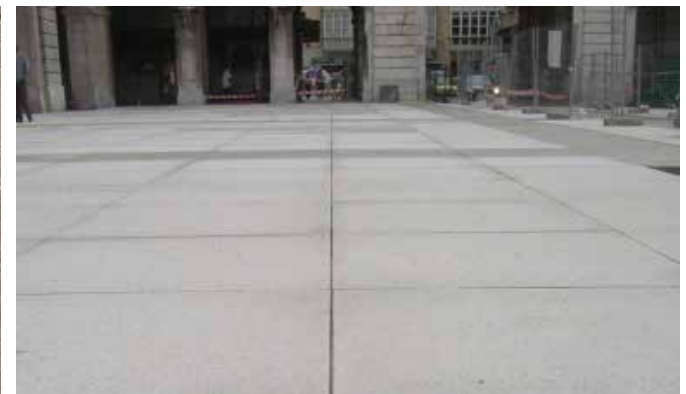
H5 Stepping stone paving
