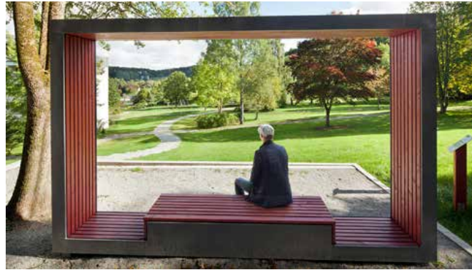
F5 Steel and timber viewing portal frame structure
