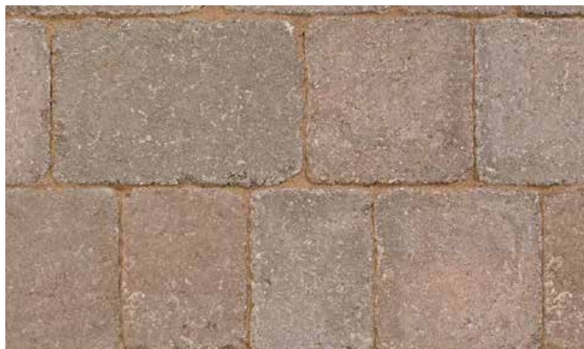
H3 'Tegula' Concrete Sett Paving
